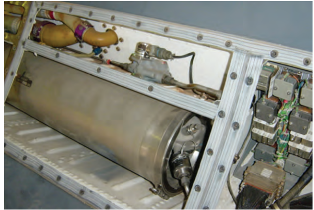
Figure 3: Airframe installation for panel 2408
