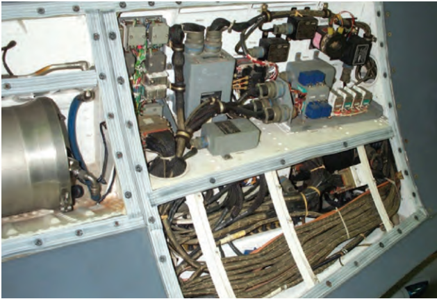
Figure 2: Airframe installation for panel 2406
